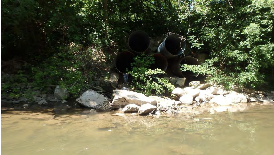
Figure 7-18: Patterson-Robbins Drain Outfall into Thames River
