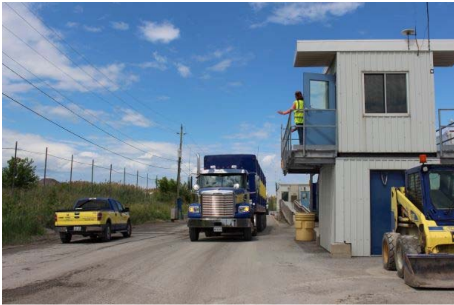
Scale house at South Landfill, Niagara Falls
