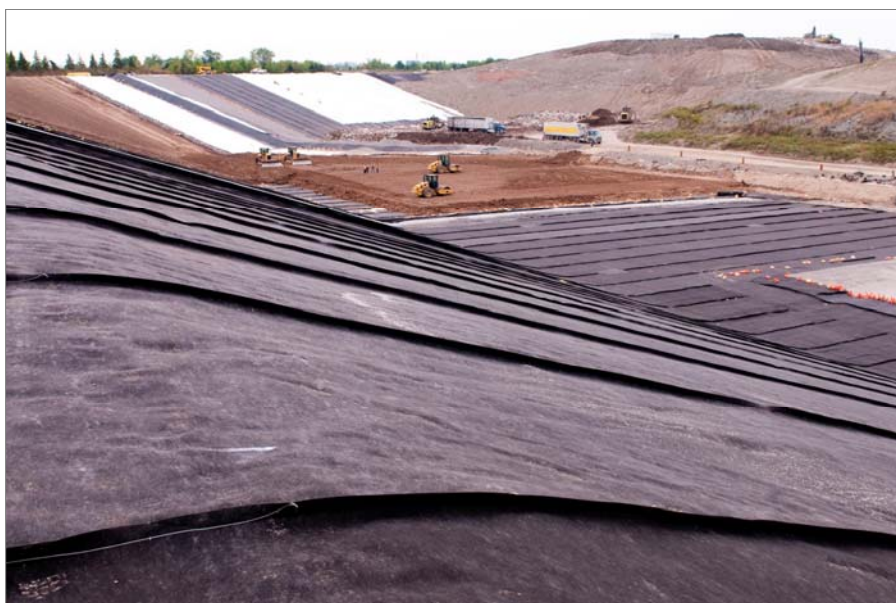
Landfill liner construction, South Landfill, Niagara Falls
