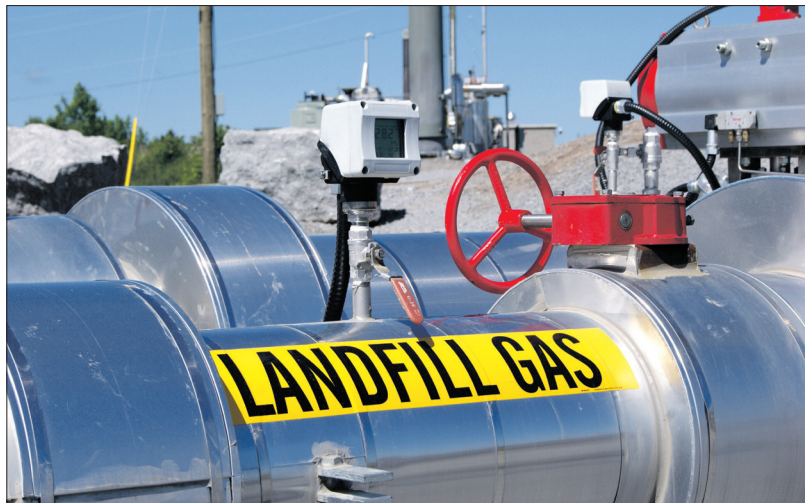
Walker South Landfill - Landfill Gas Pipeline to Nearby Industrial Energy Users
