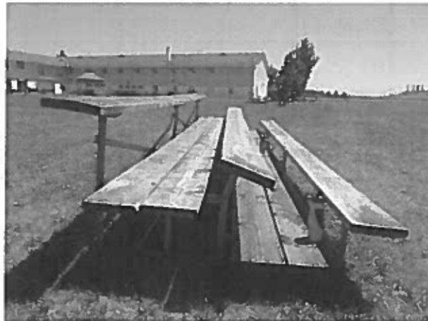
BENT STRUCTURAL FRAME (SEATING)
