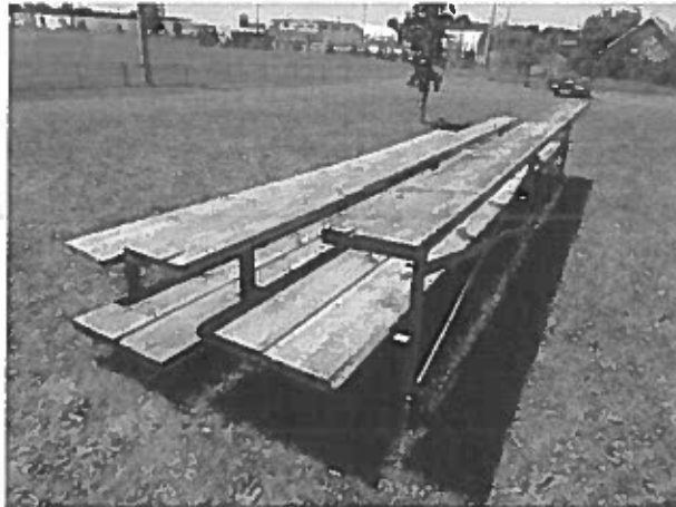
BOLT PROTRUSION, BENT CROSS BRACING, SLIVER POTENTIAL
