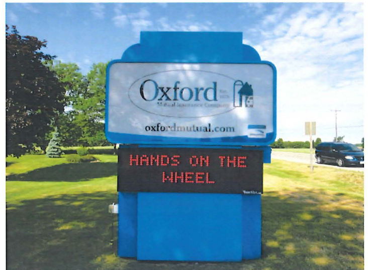
Oxford Mutual Insurance - Thamesford, ON Retro fit LED display, repair and repaint existing sign
