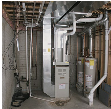
Rough-in for Mechanical Systems
