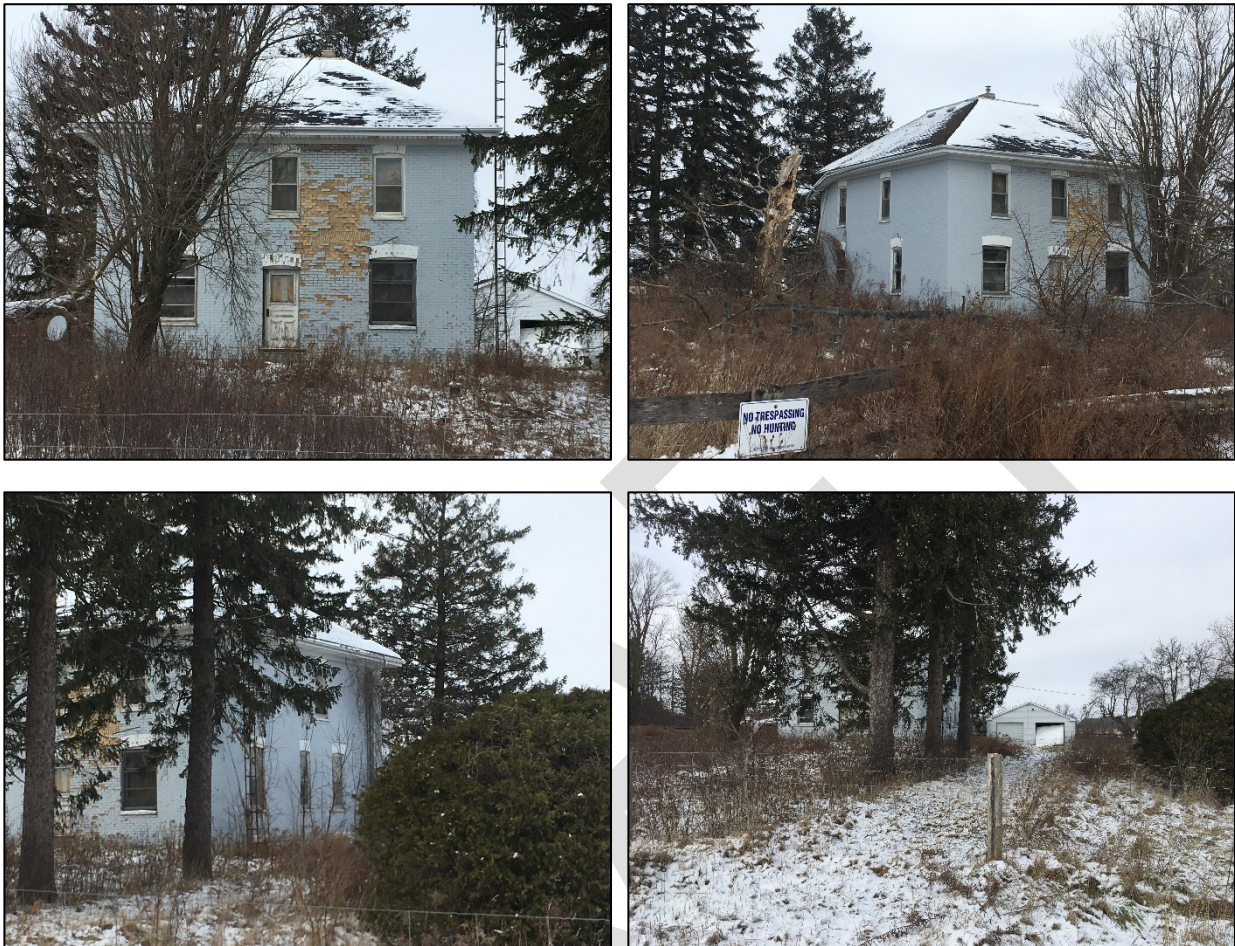
Photos 1-4: Views of front, east and west dwelling facades, as well as contemporary garage – now removed ( source : MHBC, 2019)
