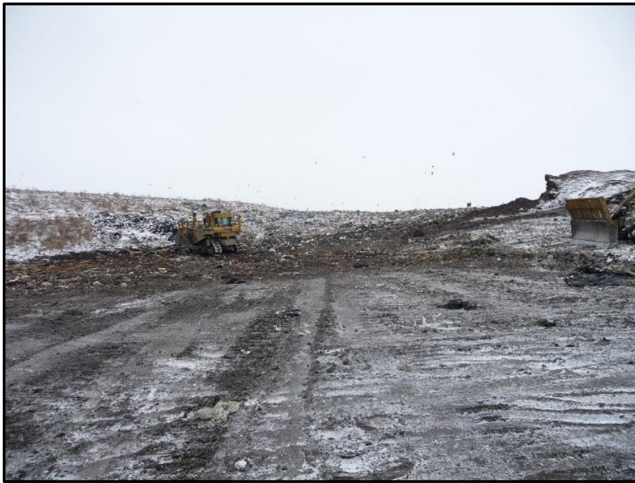
Photograph 4. Tipping Face of the Stratford Landfill March 28, 2018
