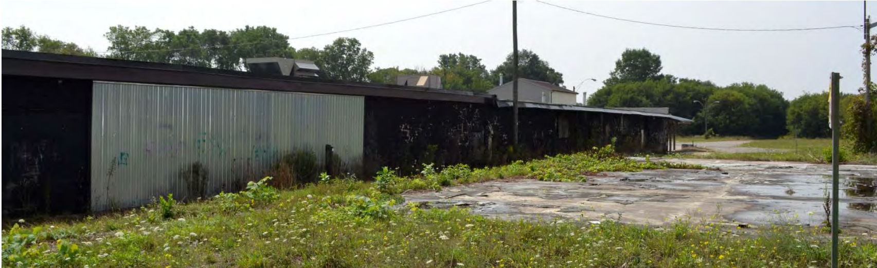
Figure 3- Northern limit of existing building (facing south west)
