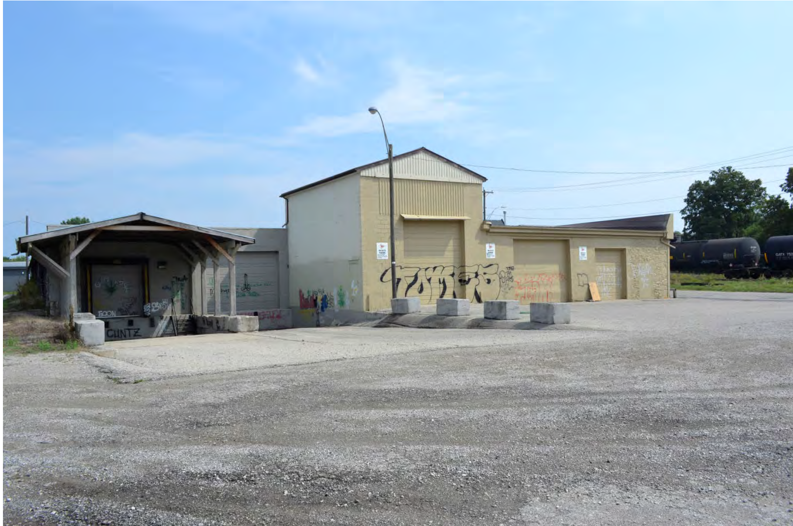
Figure 2 – Rear of Existing Building (facing east)
