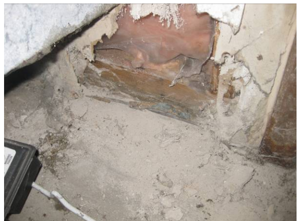
Photo 10 - Mech'l room (drywall removed)
