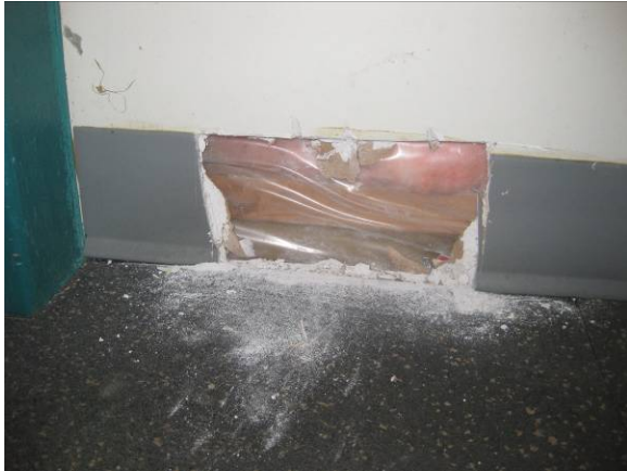
Photo 7 - Change room (south) wall
