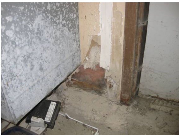
Photo 9 - Mech'l room (drywall removed)
