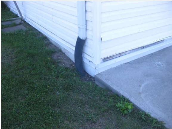
Photo 19 - Connected downspout
