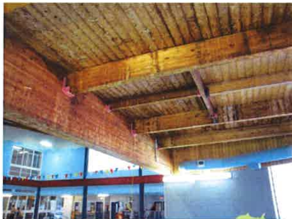
Fig. 1 – Wood beams in pool area appear to have some mold on the surface.
