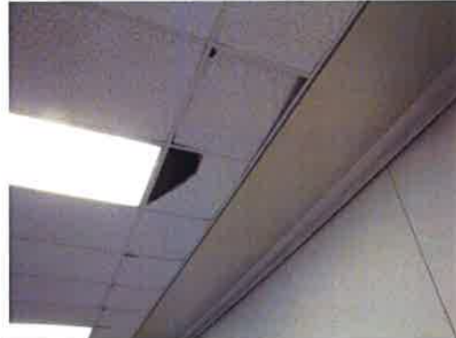
Figure 10 - Damaged ceiling tiles
