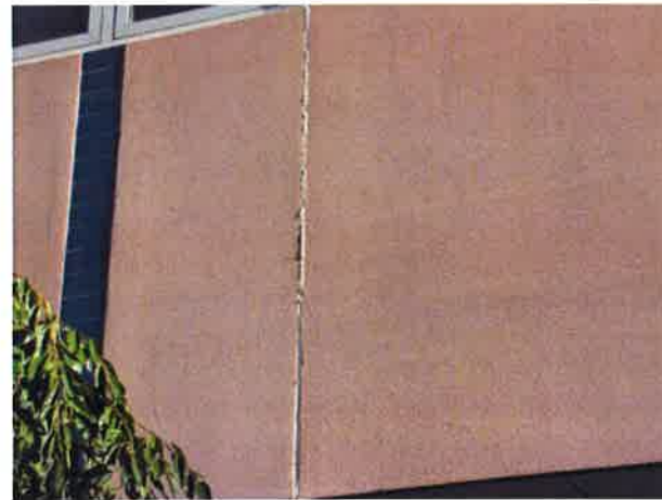
Fig. 6 – Outsulation (EIFS) poor caulking installation
