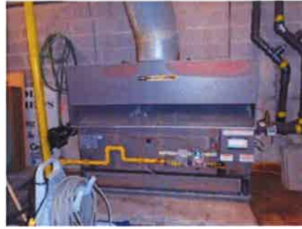
Fig.27 - Roof Mounted Down Blast Exhaust Fan | Fig. 28 - Pool Boiler (Scorch Marks on Surface)
