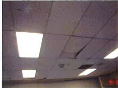
Figure 9 - Damaged ceiling tiles
