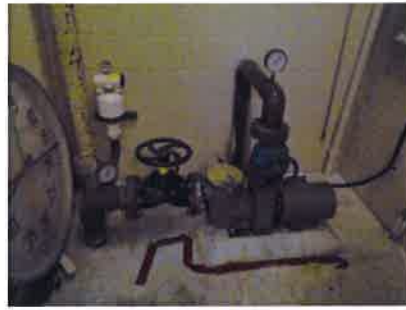
Fig. 29 - Pool Sand Filters | Fig. 30 - Whirlpool Pump
