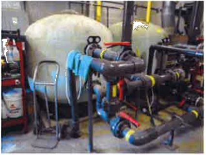
Fig. 29 - Pool Sand Filters | Fig. 30 - Whirlpool Pump
