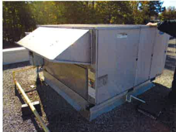
Fig. 25 - Carrier Packaged Air Handling Unit (15 ton)
