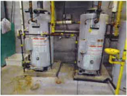
Fig. 31 - Domestic Hot Water Heaters and Storage Tank | Fig. 32 - Fire Alarm Panel
