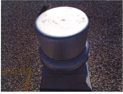
Fig.27 - Roof Mounted Down Blast Exhaust Fan | Fig. 28 - Pool Boiler (Scorch Marks on Surface)
