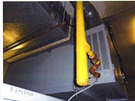
Fig. 26 - Engineered Air Pool Handling Unit (Heating Unit)
