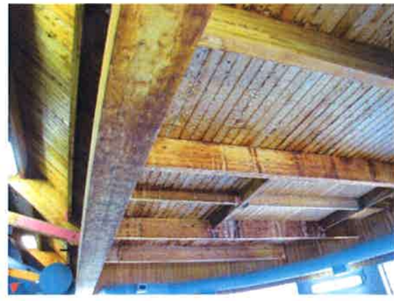
Fig. – 2 Wood beams and decking appear to be water damaged.
