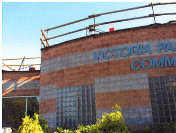
Fig. 5 – Architectural block is saturated
