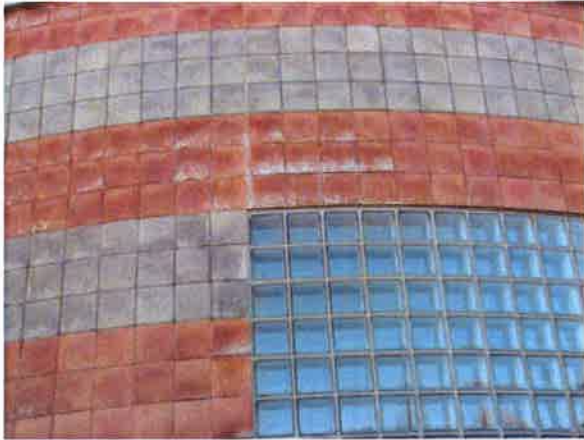
Fig. 3 – Architectural block is saturated
