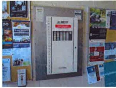
Fig. 31 - Domestic Hot Water Heaters and Storage Tank | Fig. 32 - Fire Alarm Panel
